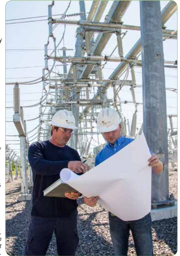
Darren Milliken, Lineworker and Erik Hall, Supervisor Substation Automation and Tech Support, review plans for upcoming work at Larrabee Road Substation in Lewiston.
