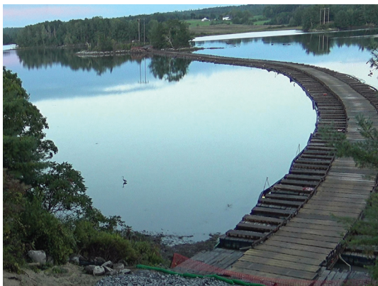
A floating road rose to the challenge of helping us to improve reliability for our customers.
