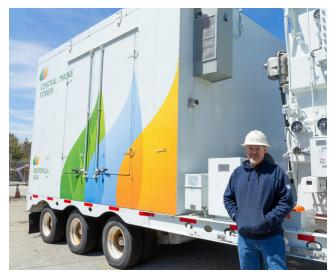
Recently, an animal exploring inside our Monmouth substation made a wrong move that resulted in a power outage. Knowing that extensive repairs had to be made before power could be restored, a mobile substation was put into place so power could be delivered to customers while our crews worked to safely restore power.
