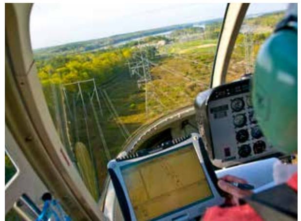
Helicopter inspection along one of CMP's transmission line corridors.
