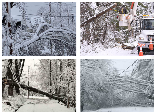
Photos taken April 10, 2020, following a storm that brought strong winds and heavy wet snow.
