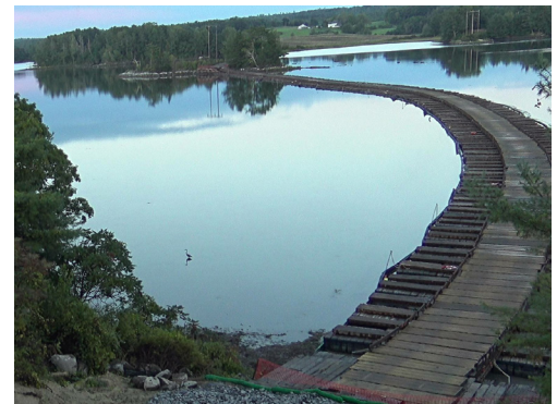
A floating road rose to the challenge of helping us to improve reliability for our customers.
