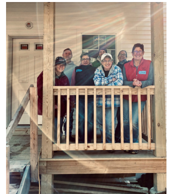
CMP volunteers helped build David and Marie's house on their team build day!
