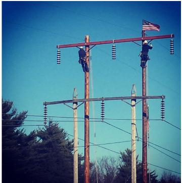
CMP will replace five structures in two communities with taller poles to comply with North American Electric Reliability Corp. (NERC)-mandated standards. The old structures will be taken down.
