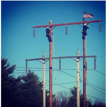
CMP will replace two structures in two communities with taller poles to comply with North American Electric Reliability Corp. (NERC)-mandated standards. The old structures will be taken down.
