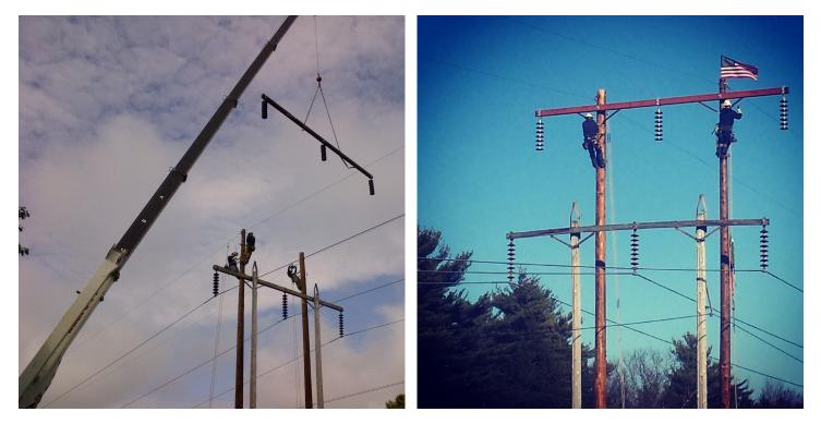
*CMP will replace 42 structures in seven communities with taller poles to comply with North American Electric Reliability Corp.* (NERC)-mandated standards. The old structures will be taken down.
