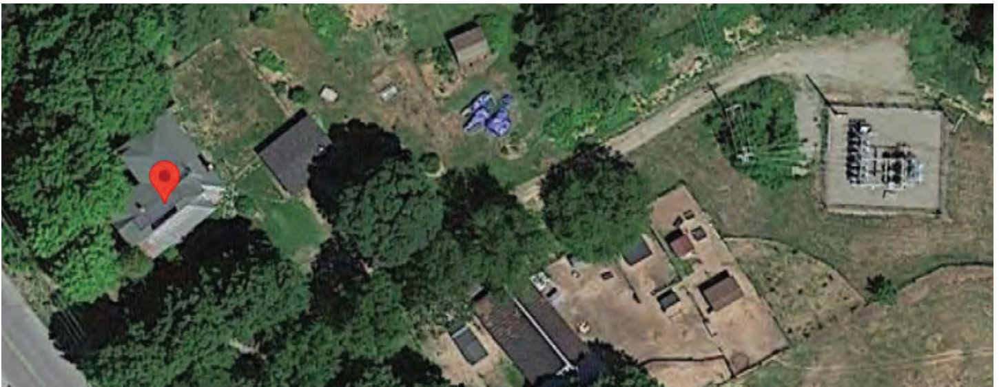
North Anson Substation, 905 River Road (Google Map View) - December 2022
